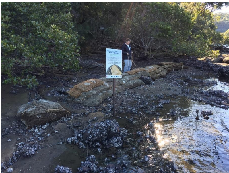
Photo 3.8. Structures installed at HD Robb Site.
