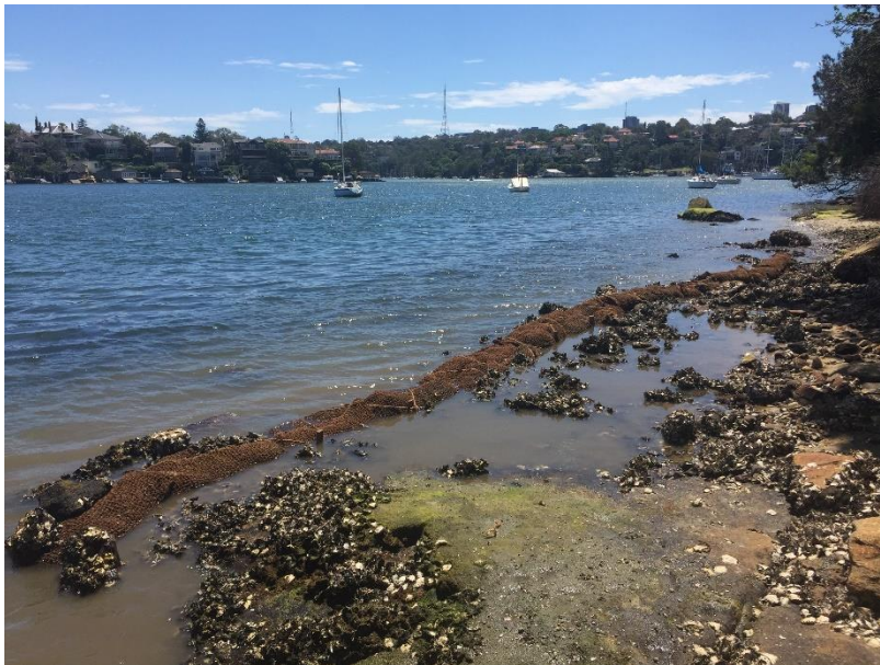
Photo 3.6 Structures installed at Greenwich Point Site.
