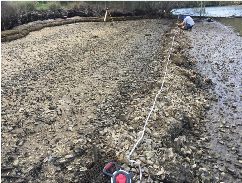
Photo 4.6. Photo taken at Sugarloaf Site showing the difference in the degradation of structures on the low-mid and high intertidal zone – April 2018.
