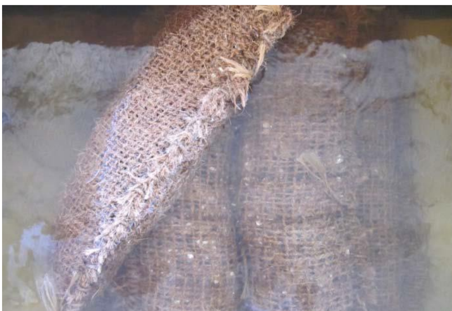
Photo 3.3. Complete displacement of an unsecured crest bag after wave attack (Coghlan 2017).
