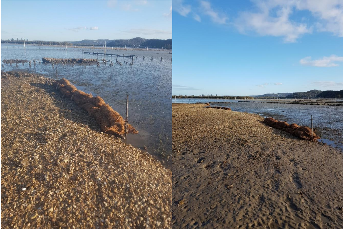
Photos 3.2.1 and 3.2.2. Living shoreline structures installed at treatment site - July 2020.
